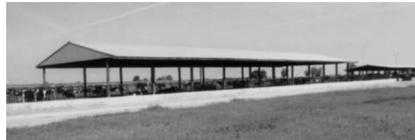
Four Sides Open, Metal on Pole Frame
