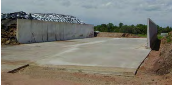
Bunker Silo – Precast Wall Panels
