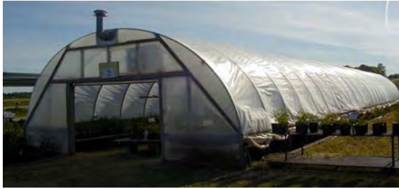
Light Pipe Arch, Wide Spacing, Polyethylene Cover
