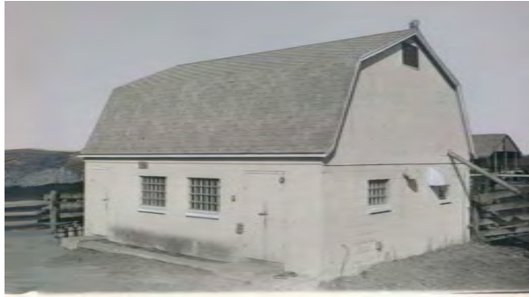
1-Story Concrete Block and Frame Milk House
