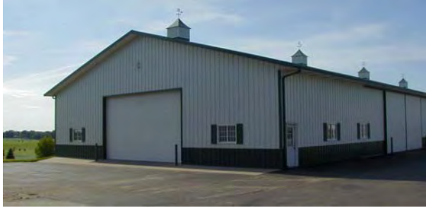
1-Story Pole Frame
