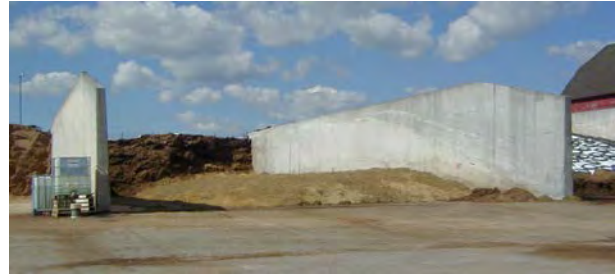
Bunker Silo, Concrete Walls
