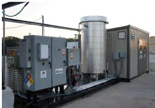
BIO CNG System CNG Pumps
